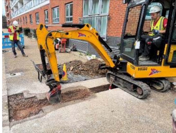
The work to install the electricity bollard at Wolverton. See opposite page and back cover for more details
