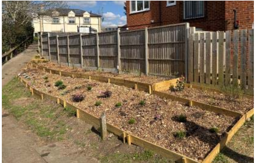
The finished raised beds, newly planted
