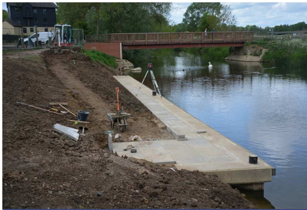
Phase 2 in progress
